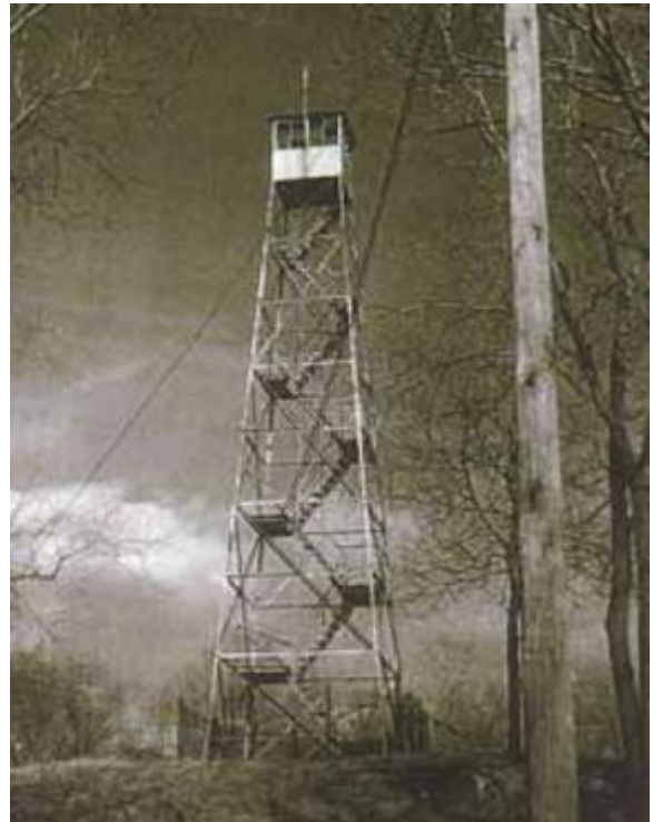
Fingerboard Mountain Tower
