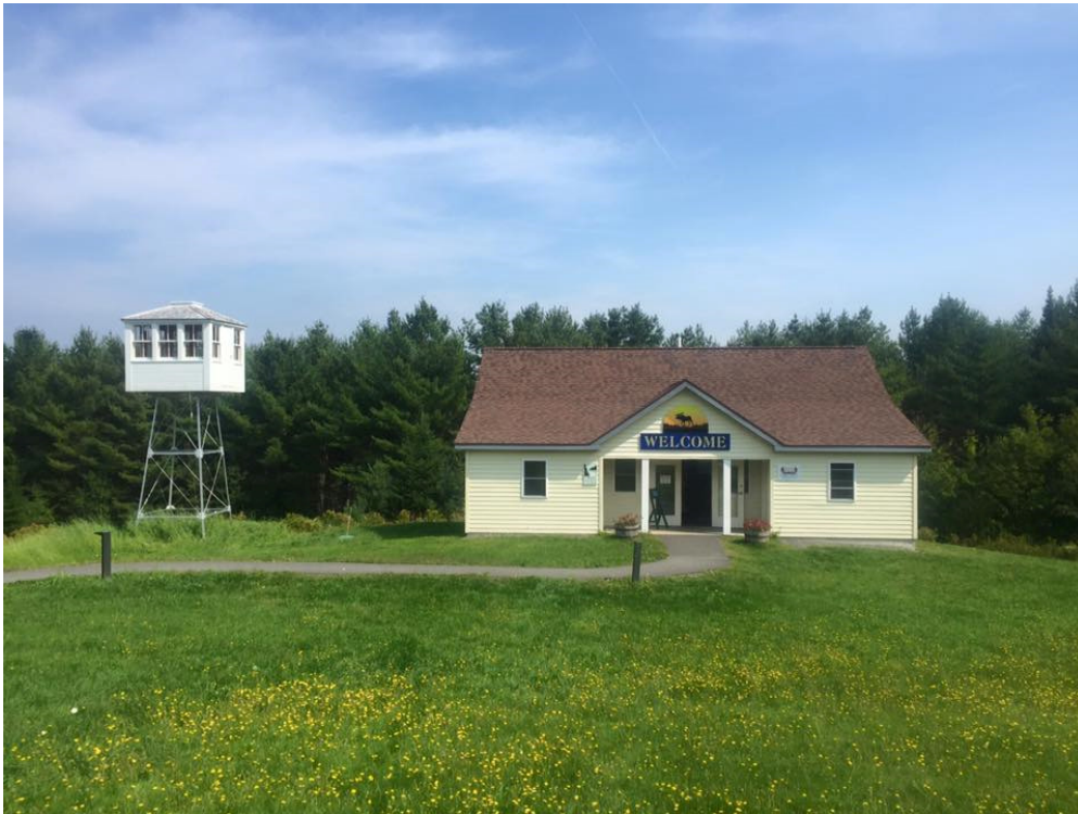
The former Squaw Mountain fire tower is now erected at the Greenville visitor center using the original 1919 restored steel and rebuilt cab.
